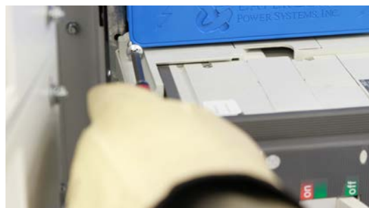
Screws Help Secure The Breaker
